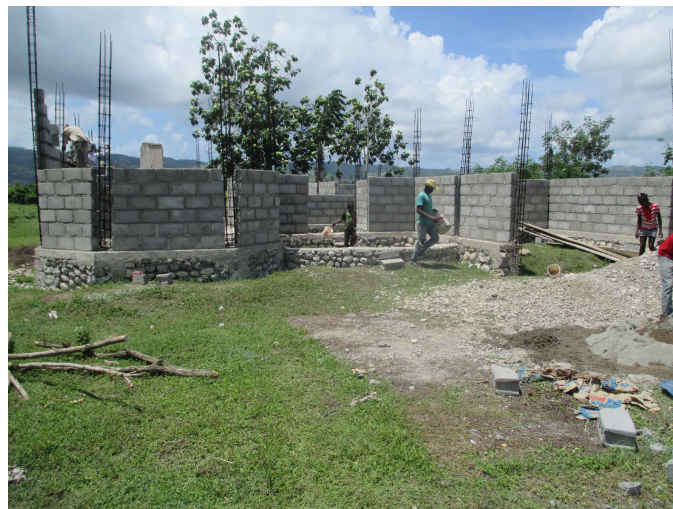
Figure 5 Building house for Pastor Prince and family of 6.
