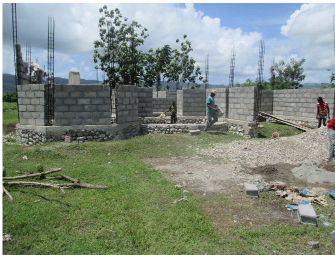
Figure 6 Building house for Pastor Prince and family of 6.
